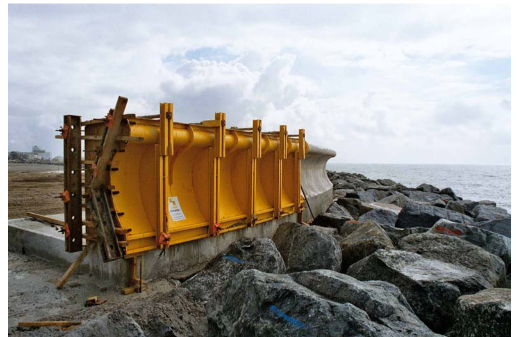
SEAWALL FORMWORK
