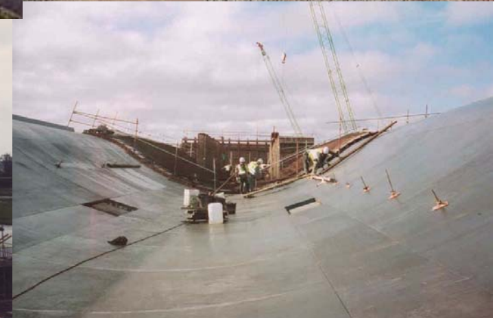
PUSH LAUNCH ~ BRIDGE CONSTRUCTION
