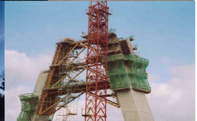
FALSEWORK for BRIDGE CONSTRUCTION
